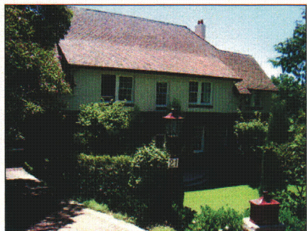
Figure 2.38 No. 21 Lorne Avenue, Killara.
